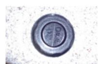
Open air control fittings when in HIGH speed Jets mode to provide air mix to jets. On/Off Toggle.
